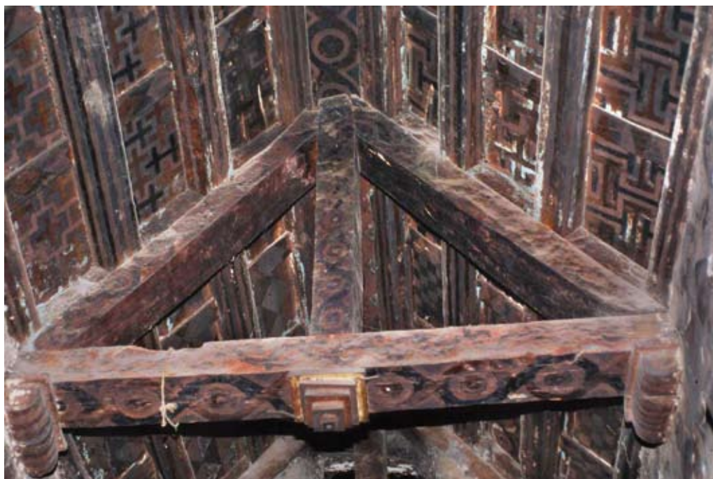
13. ጌጳጳክና ጳጳጳክና ልጳጳጳ church, kingpost, tie beam and principal rafters supporting saddle-back roof
