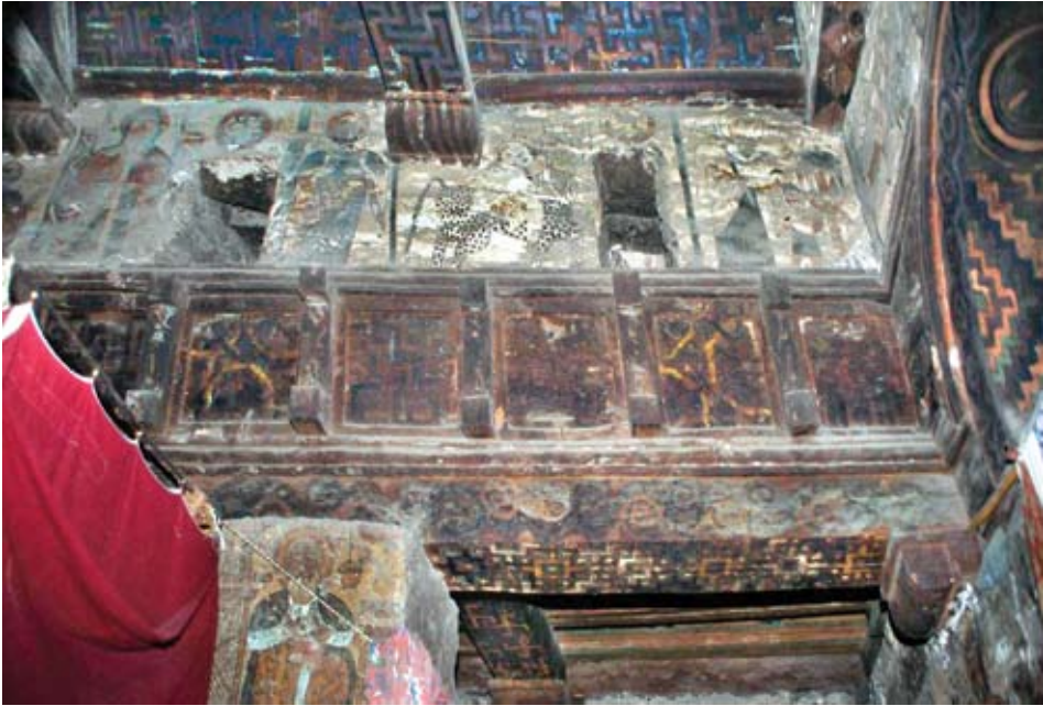
9. Զմակինա Մաժինե Ալամ church, northeast corner showing pillar, principal beam, frieze, and clerestory ceiling timbers above the nave
