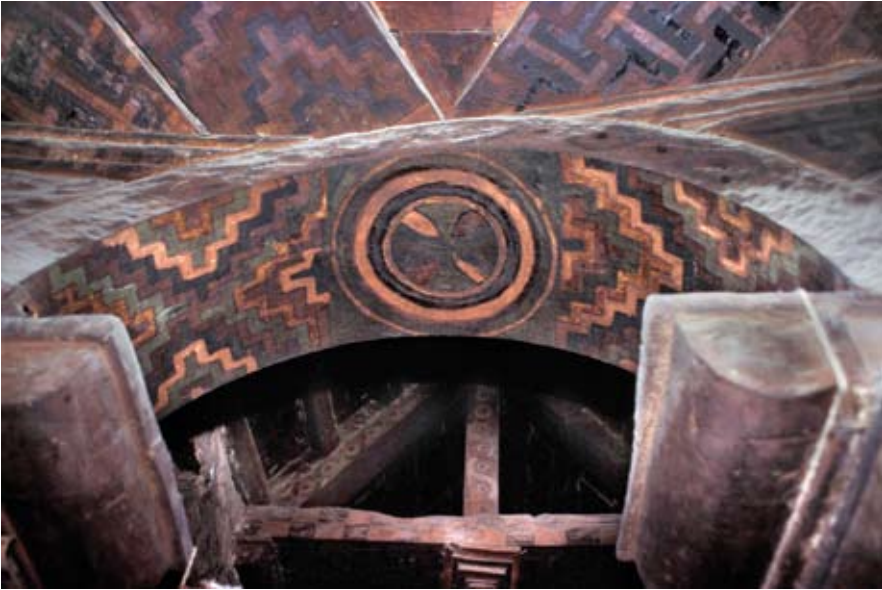
11. Ēmäkina Mādḡane Alām church, sanctuary arch facing west
