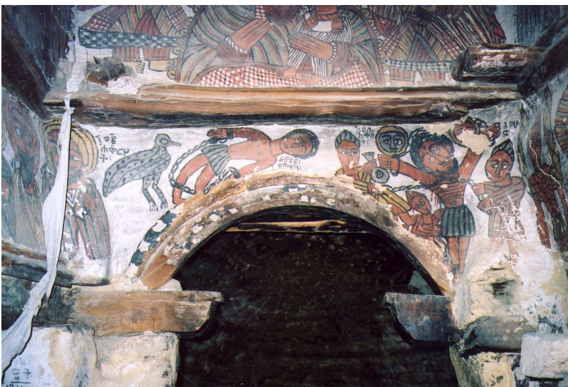
Large painted surfaces with paint falling off.
